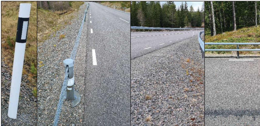
Figure 11: Existing infrastructure other than road signs which were investigated. Left to right: reflective poles, cable crash barriers, classical w-shape crash barriers and pipe crash barriers.
