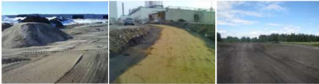
Figure 3. External recycling of foundry sand. Left: Use of foundry sand and cupola furnace slag as fill material at Volvo in Skövde. Centre: Foundry sand in pipe trenches at Scania in Södertälje. Right: Sand from Arvika foundry used as landfill material.
