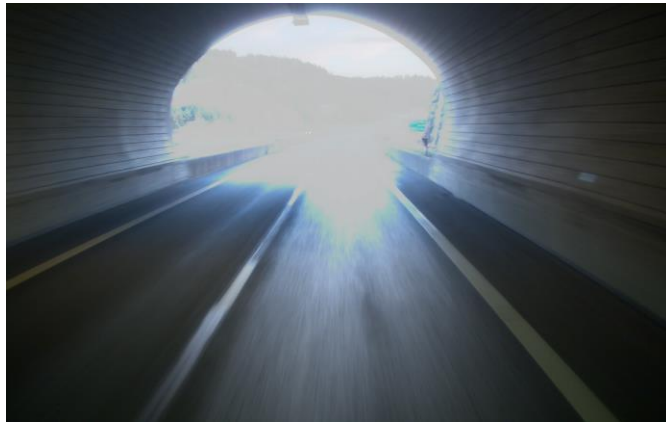
Figure 1 A tunnel exit found along highway in southern Sweden
